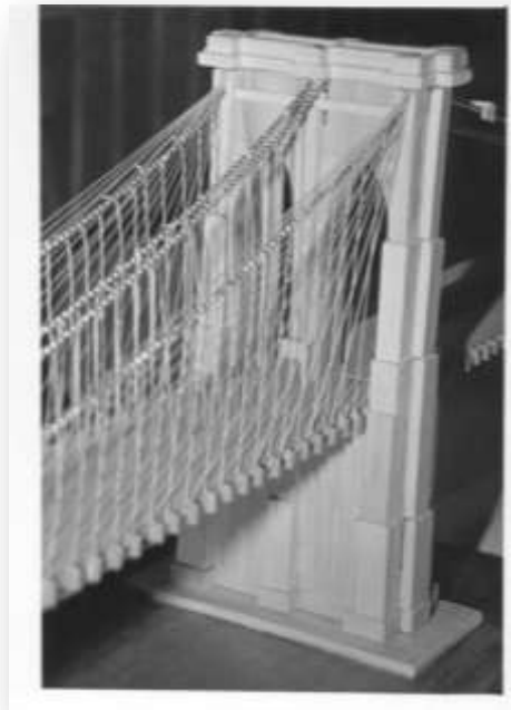
Figure 6. A model of the Brooklyn Bridge. The vertical stays carry the entire stress of the roadway.
