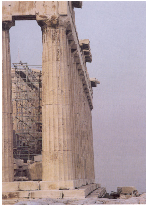
Figure 6. The Parthenon curvature along the northern steps.
