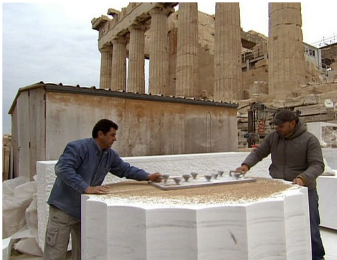
Figure 5. The ancient method of grinding columns with sand and a grinding plate can be precise up to one twentieth of a millimeter. (Secrets of the Parthenon homepage/ NOVA homepage.)
