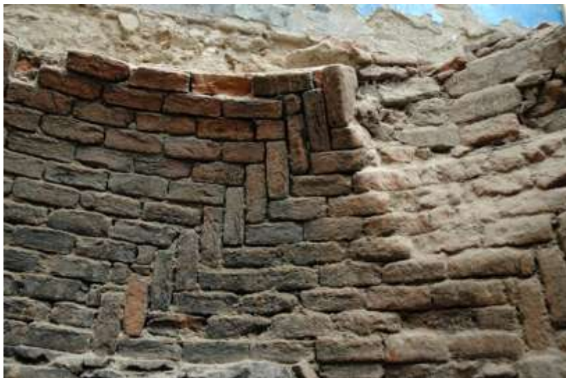
Figure 1 The Herringbone pattern of bricks in Brunelleschi's recently discovered original model of the Cupola. http://news.discovery.com/history/archaeology/scale-model-discovered-for-florence-cathedral-130110.htm
