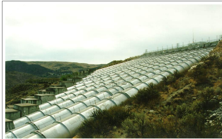
Twelve Discharge Pipes from Lake Roosevelt to Feeder Canal
