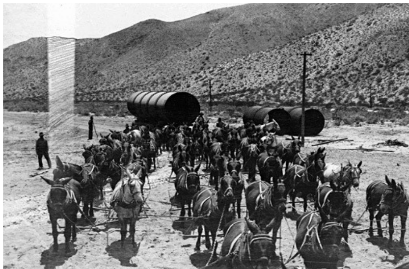
Mules haul pipe for Jaw Bone siphon
