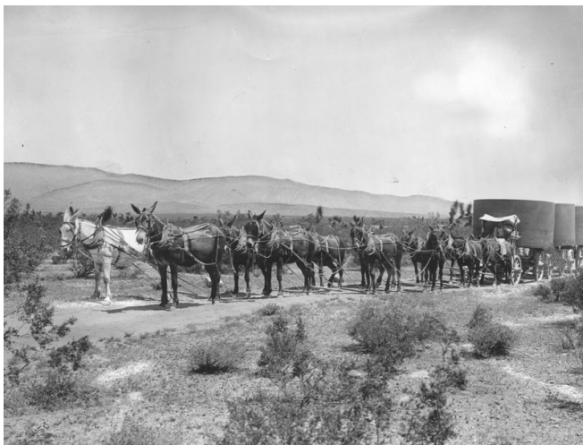
Mule team hauling materials to build the Los Angeles Aqueduct The roadless territory was too tough for the automotive travel of that era
