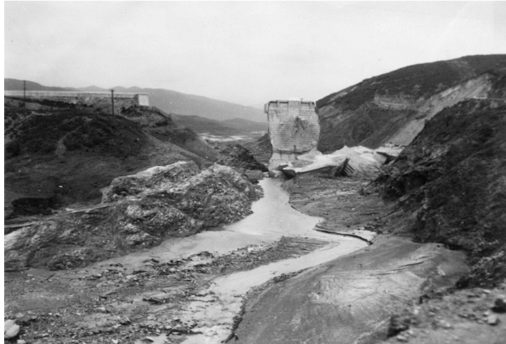
Saint Francis Dam, after its collapse
