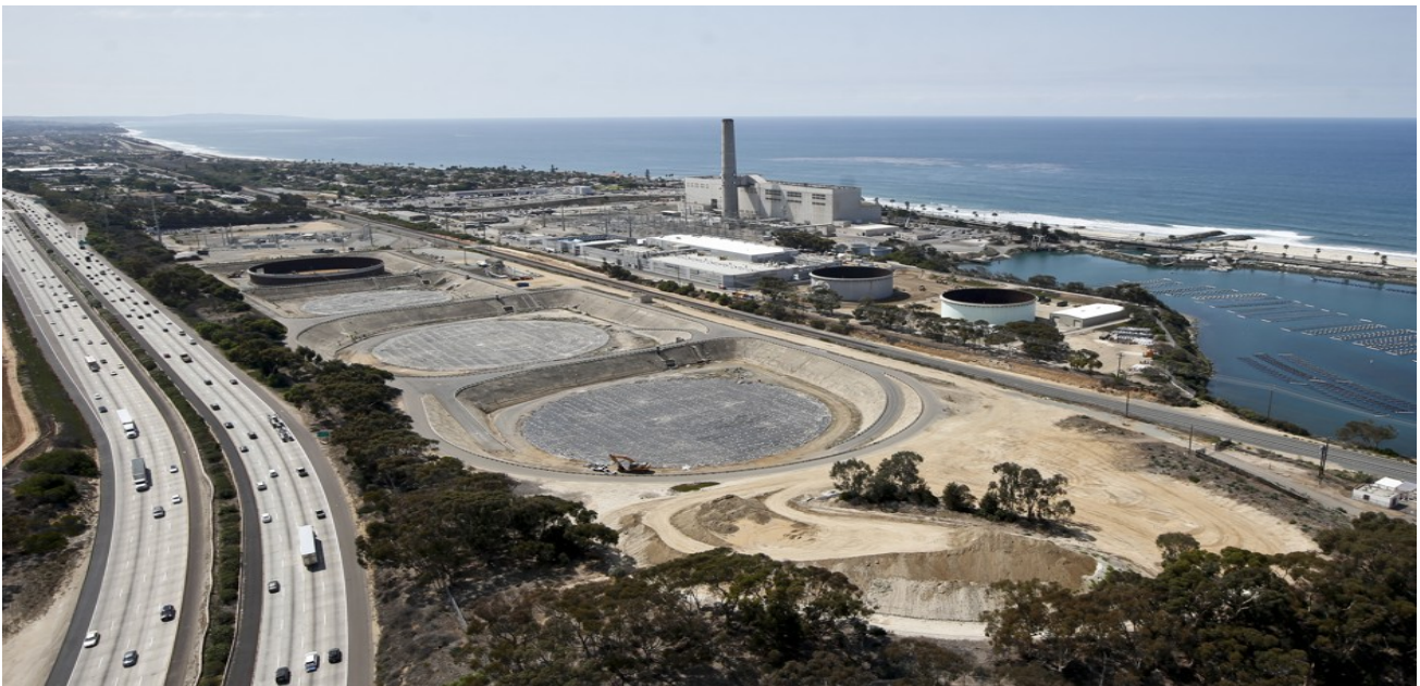
The desalination plant borders Interstate 5 on one side and the Pacific Ocean on the other. (AP Photo/Lenny Ignelzi)
