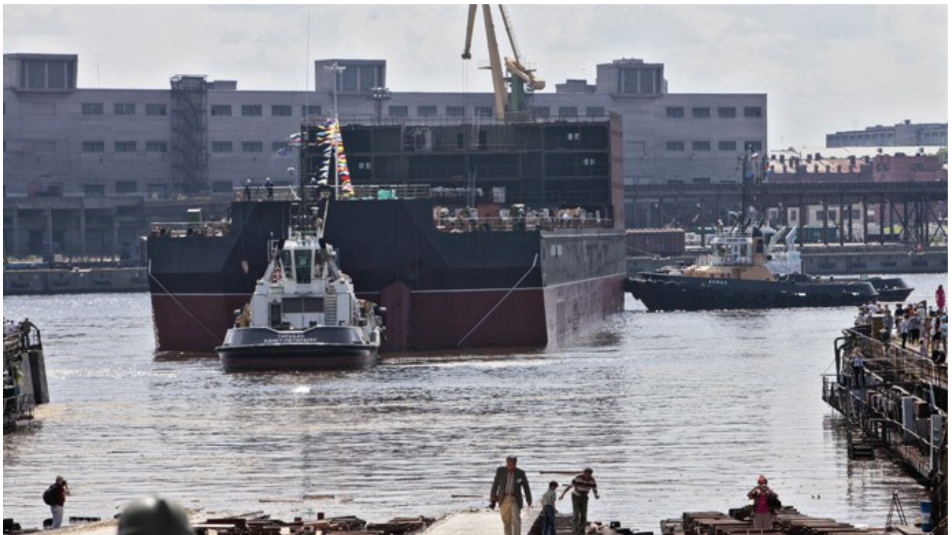
Russian floating nuclear powerplant “Academic Lomonosov” under construction
