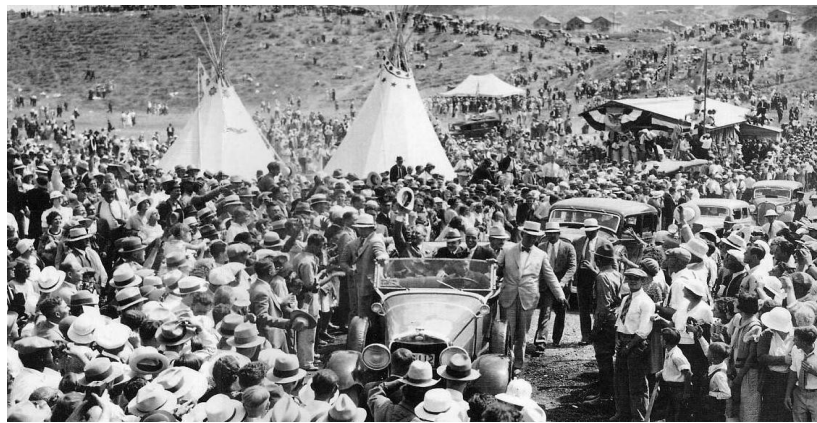
20,000 Greet FDR at Grand Coulee Dam 1934
