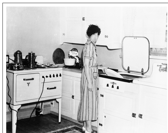
The farm kitchen after electrification
