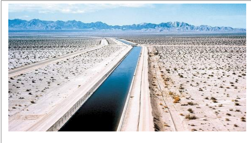
Figure 46) The Colorado River Aqueduct
