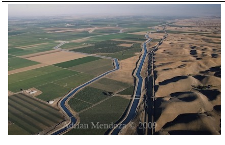
Figure 37) The California Aqueduct
