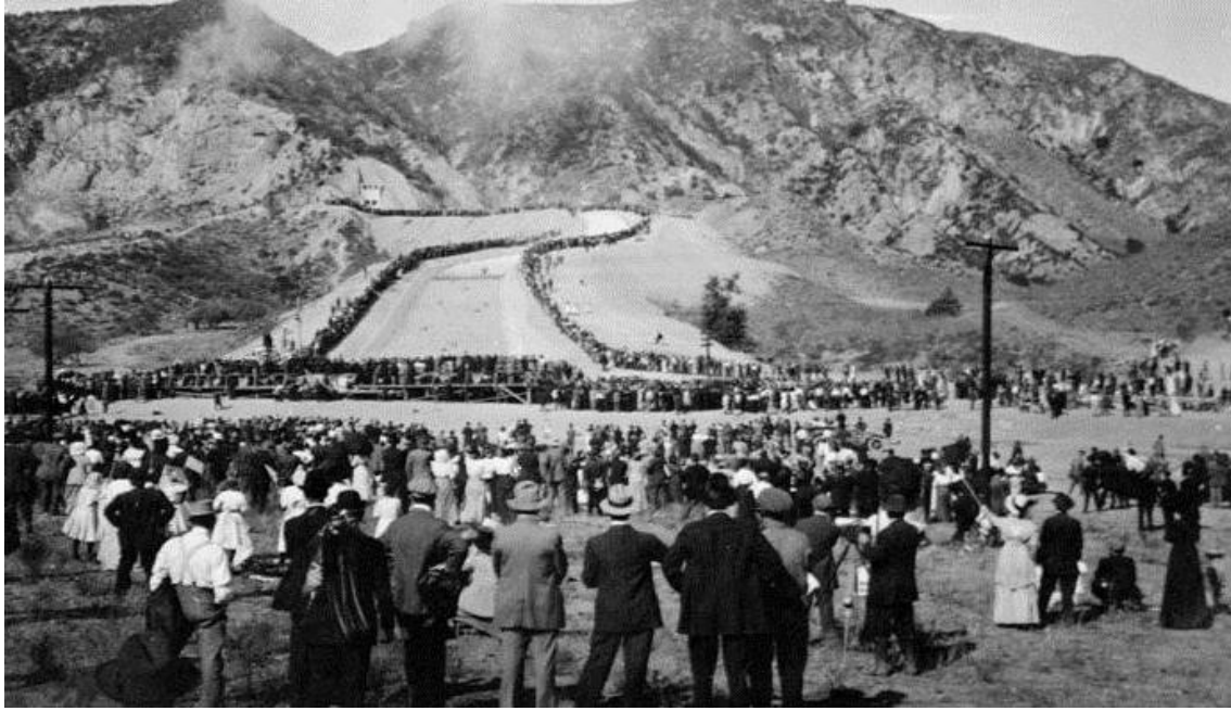
November 5, 1913 - The water gates are opened and the Los Angeles Aqueduct water starts to flow down into the San Fernando Valley
