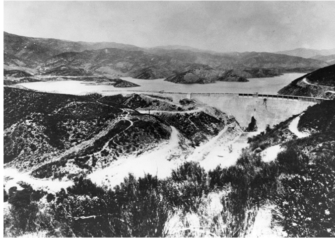
Saint Francis Dam-- shortly before its collapse
