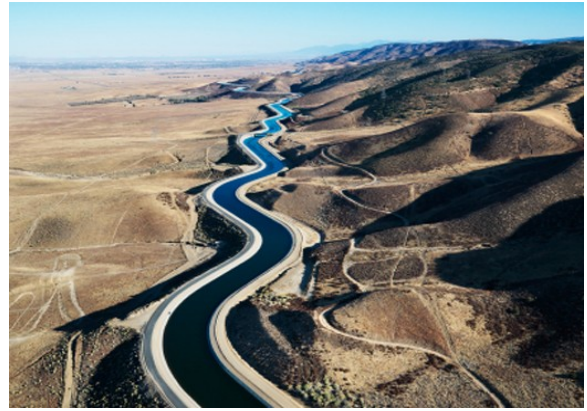
The California Aqueduct
