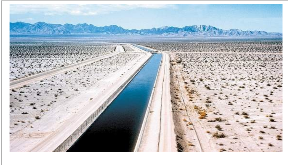
Figure 46) The Colorado River Aqueduct
