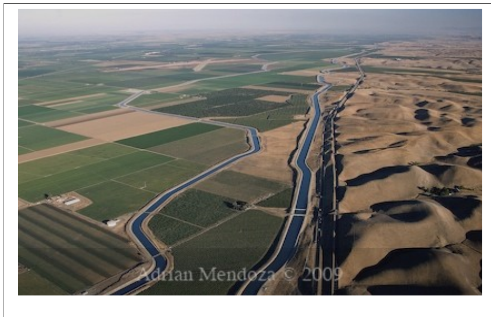
Figure 37) The California Aqueduct
